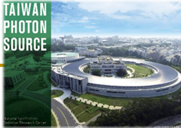
Used in the storage ring of accelerator
